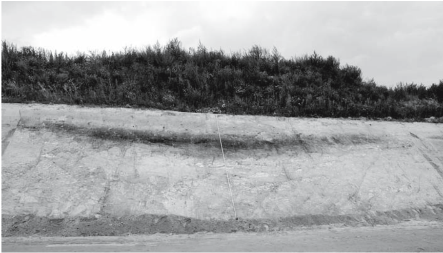
Fig. 4. A fossil closed depression at Kolonia Dąbrowica, exposed in the road cutting within the Lublin Ring Road under construction (July 2012)
